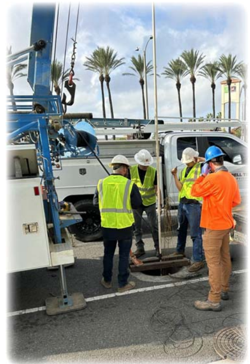
Rehabilitation Conducted on a Monitoring Well
